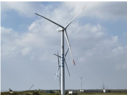
Figure 1 The wind turbine
